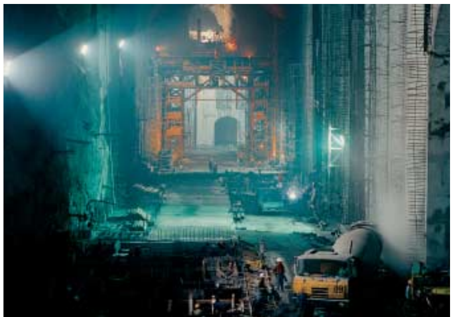
Concrete works in powerhouse cavern
