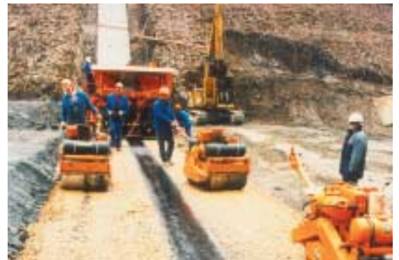
Construction of asphalt core in rockfill dam
