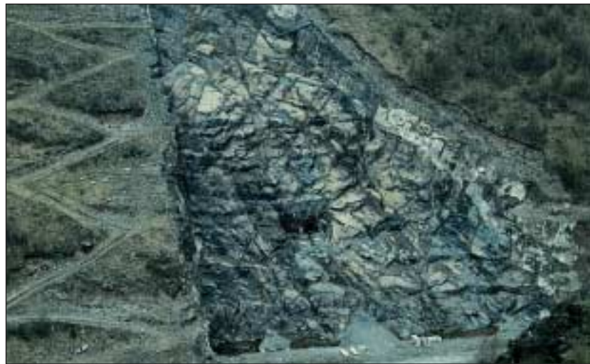
Foundation excavation for concrete gravity dam
