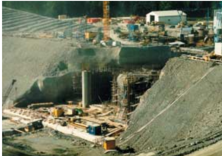
Rock excavation for intake structure
