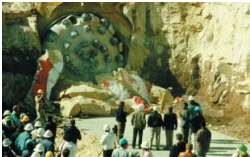
Break through of TBM
